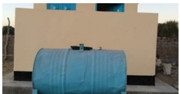
Panthou PHCC Latrine rehabilitated by IHO
